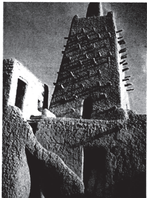
Source 5: Mosque of Djingereyber, Timbuktu
